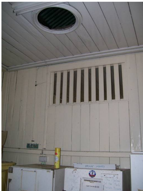
Figure 53 Photo showing slatted high level opening between R2 and R3. This photo also shows the ceiling rose missing in R3 and the mortise in the rail of the single skin wall for the power to come down to the power point above the fridge.
