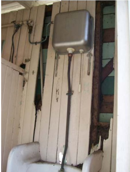
Figure 64 (above left) Note extensive termite damage to southern wall of lavatory block
