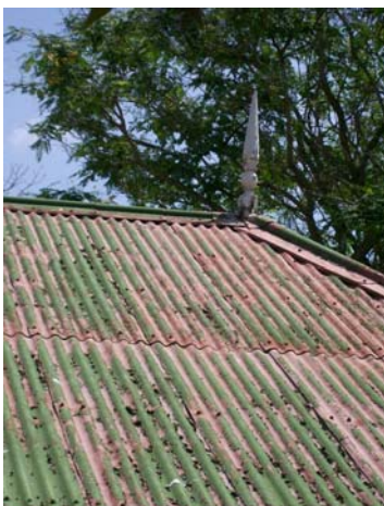
Figure 61 Roof at front showing finial and sheeting
