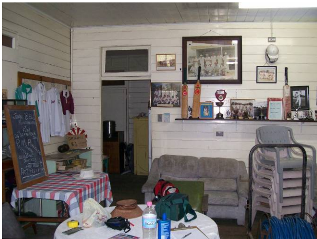
Figure 50 internal elevation towards the south in R1 showing D9, including fan light. This door probably incorporated a four panel door leaf.
