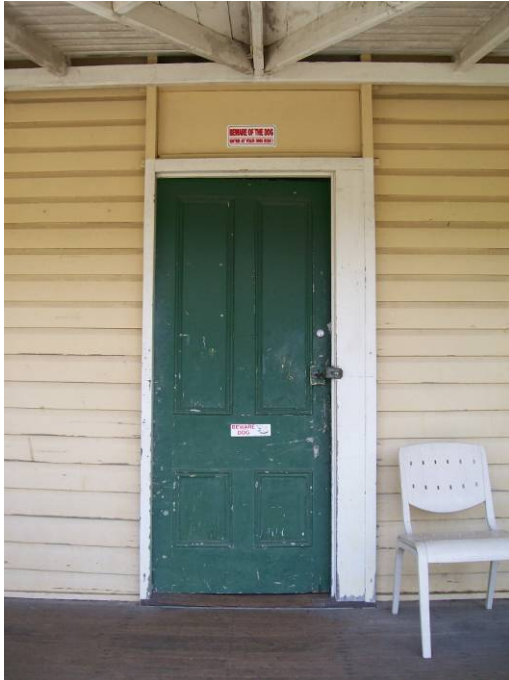
Figure 47 Example of tusk tenon jointed framed door opening onto the verandah reduced for a 4 panel door. This would have original been a set of French doors with a fanlight.
