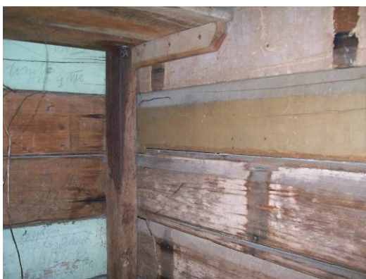
Figure 46 Photo showing underside of timber shelf in R6 and recycled chamfer boards
