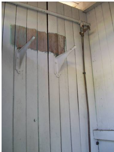
Figure 58 Location of previous high level cast iron cistern in ladies.
