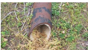
Figure 28 Drain discharging low in the bank to side of concrete stair
