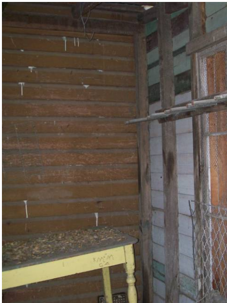
Figure 38 Photo inside the toolshed showing second hand material and dado paint stripe from a previous location. The tall window sashes on the right have also been recycled. This photo also shows the brown colour (possibly red oxide) on the northern wall inside the toolshed.
