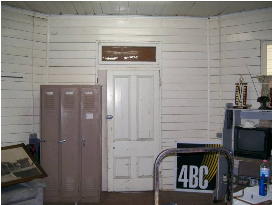
Figure 40 Photo showing internal elevation to the north inside R1. The four panel door has been recycled in the opening originally intended for French doors. The fanlight is original.
