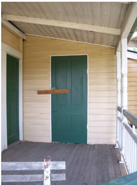
Figure 42 Photo showing raking verandah ceiling, hardwood tongue and groove floor and D4 into R9. To the right the French door opening survives.
