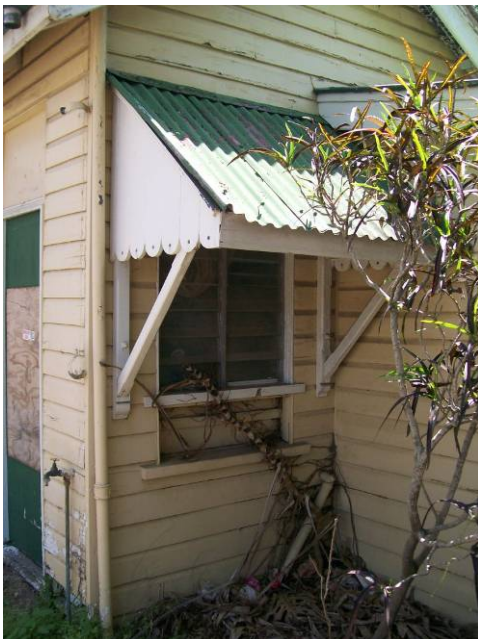
Figure 51 Elevations of W4 (above left) and W7 (above right and below left) and photo showing perspective view of hood to W7. Both W4 and W7 have original external hoods. Note W7 has original sill.
