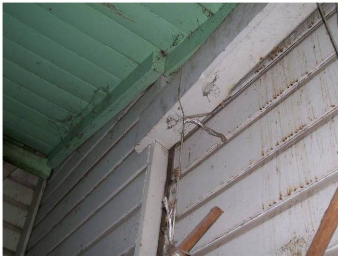
Figure 35 Joint and end of stop chamfered verandah beam still present inside the enclosed verandah store R9 at the back of R4.
