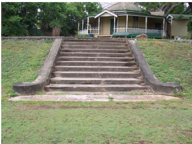
Figure 20 Photo showing concrete stair with rendered dwarf walls in the south corner of the recreation ground. It is similar to the one that stood on the previous site but has two more risers.
