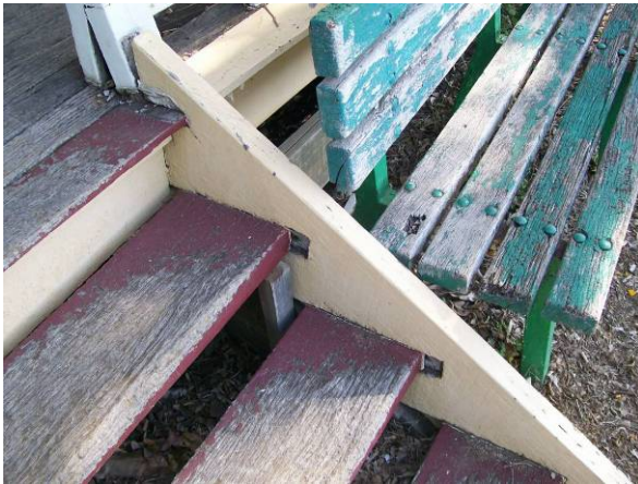
Figure 37 Photo showing replace stair treads at the front entry
