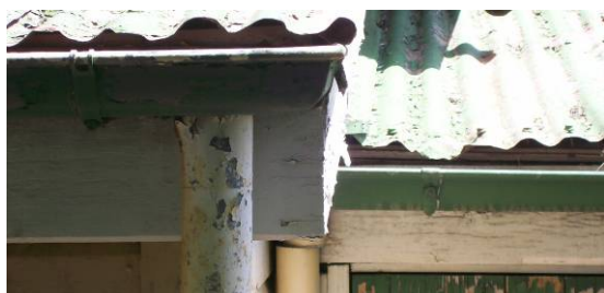
Figure 31 Photo of quad gutter showing two different types of gutter brackets
