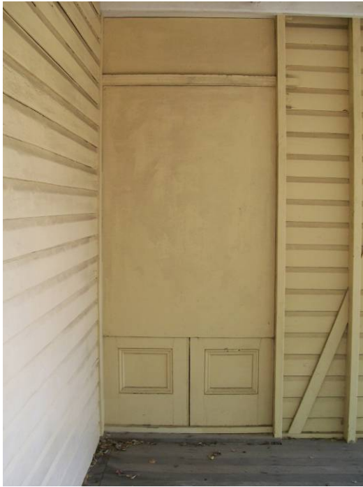
Figure 49 Elevation of D1, French doors that have been boarded up.
