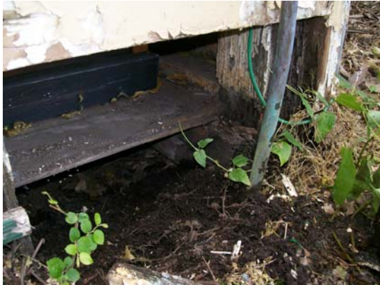
Figure 62 deteriorated bottom plate at the south
