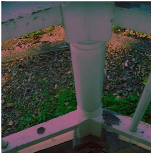
Figure 36 turned timber verandah posts. The fillets around the bases are not original. The faceted surfaces in some areas suggest they may have been hand finished although this may also be the result of subsequent refinishing.
