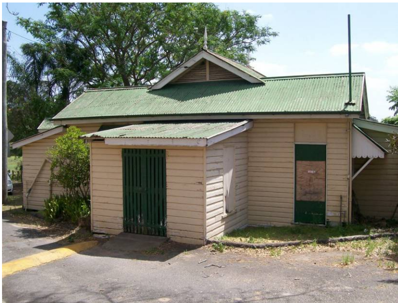
Figure 33 The southern elevation of the cricket pavilion, showing two parts of the roof meeting and the triangular vent as well as the lean-to additions. The lean-to on the left is the shower room that shows on photographs as early as 1911. The lean-to addition in the foreground is the toolshed and dates to 1913. The lean-to addition on the right shows on the historical block plan from 1936. None of the lean-to additions show in the building outline on historical site plans from 1909 and 1896.
